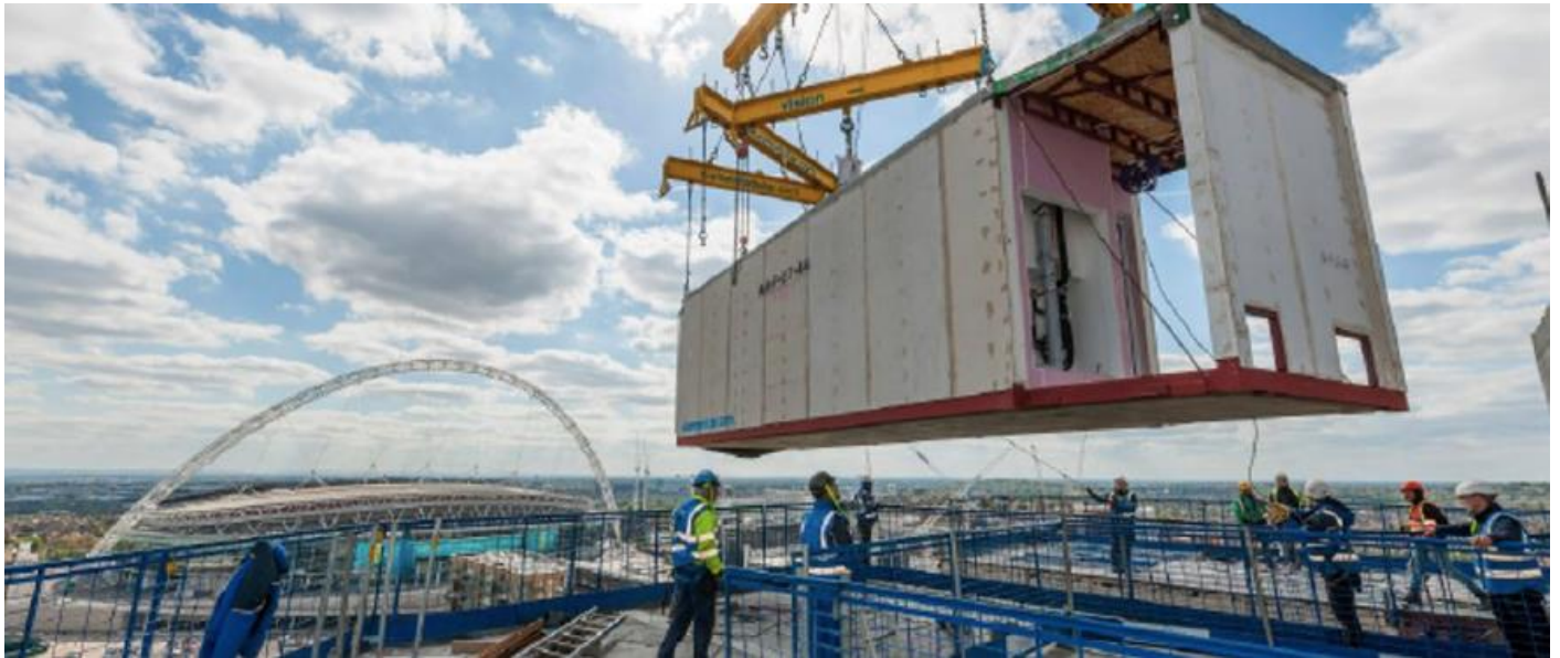
Figure 1.1 3D volumetric modular construction (MMC Category 1) - Source: https://visionvolumetric.co.uk/project/scape-wembley
