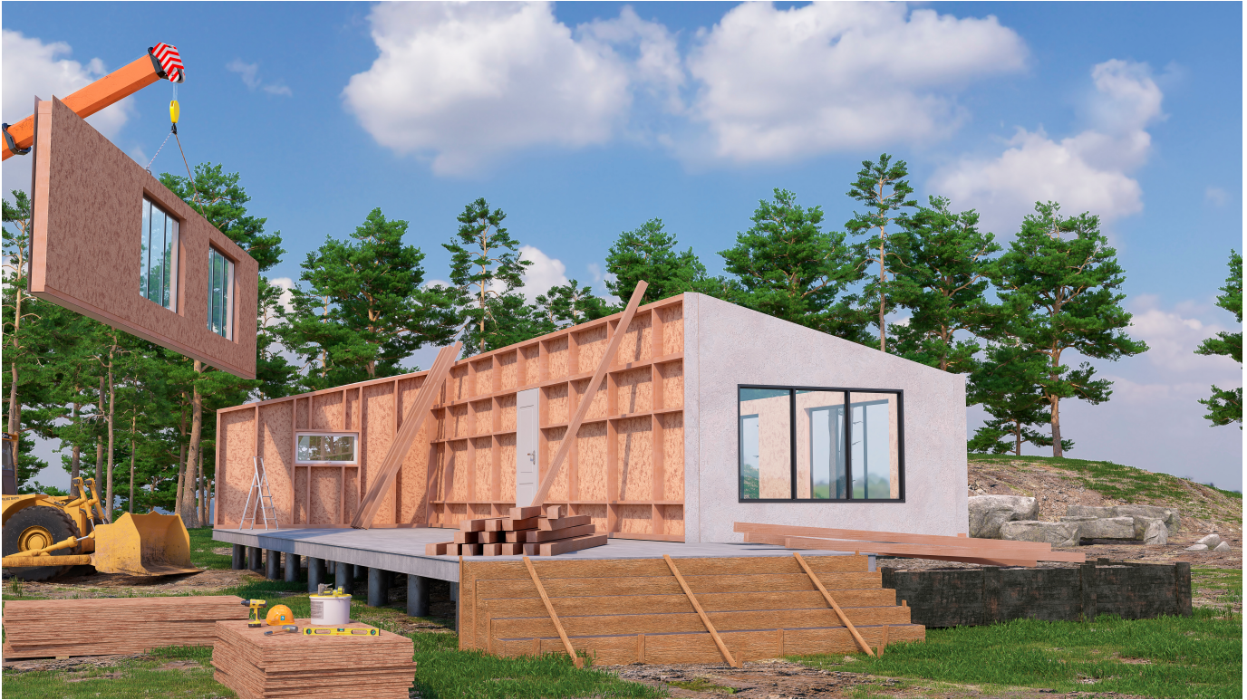
Figure 2.1: 2D panelised construction (MMC Category 2)
